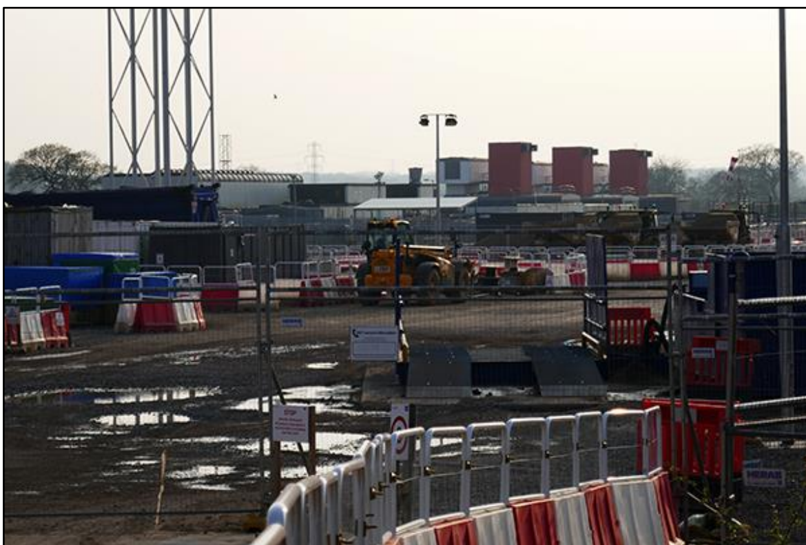
National Grid gas compressor station
