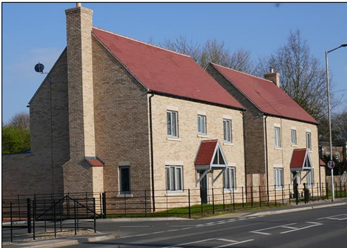
Development of two new homes on the Lincoln Road
